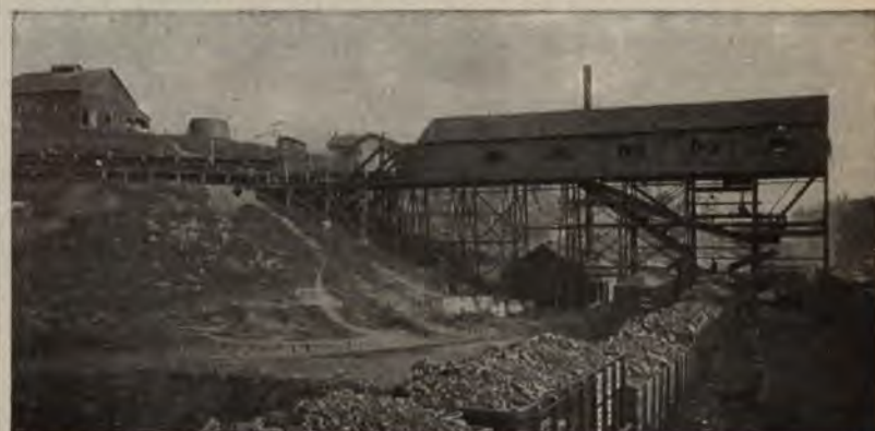
A coal breaker in West Virginia. The coal comes from the mines in masses of varying sizes. It is here crushed, cleaned, and graded in sizes. It then drops into cars which carry it to market.
